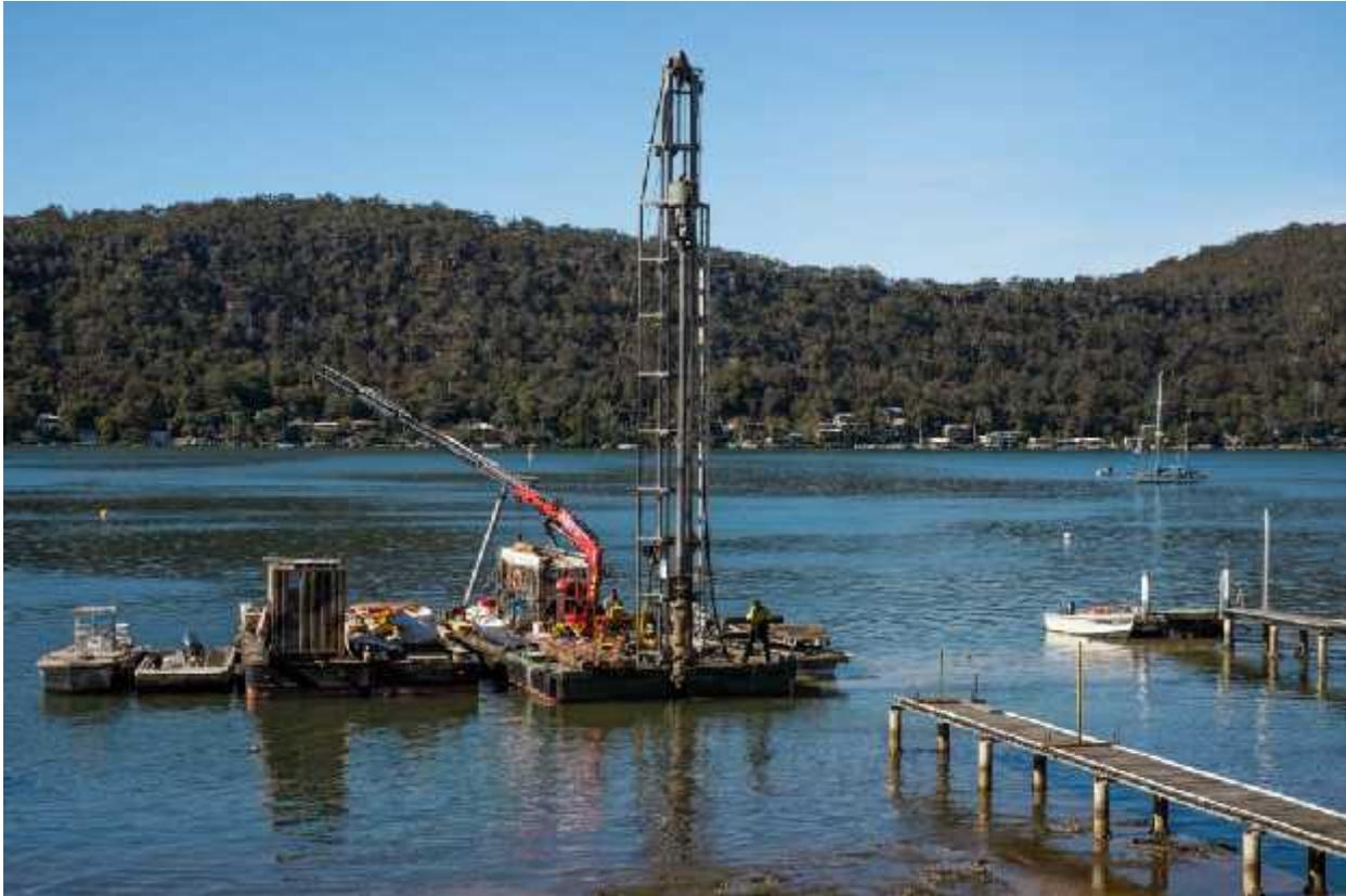
**Figure 2.8: Pile Driving Frame for Project Requirements**
