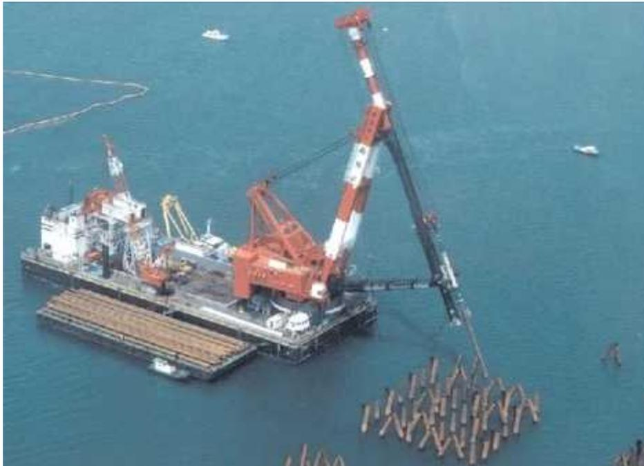
Figure 2.7: Floating Pile Driving Frame through Barge
