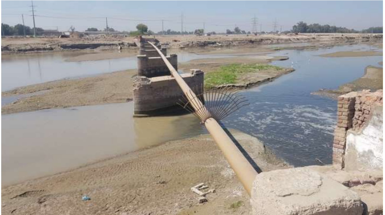
Photo 2.1: Gas Pipeline crossing (RD 16.2)
