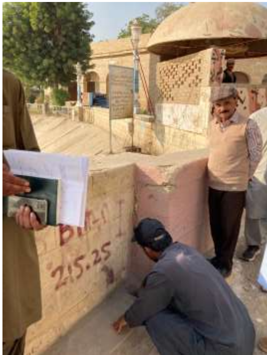
Photo 3.1: PBM1 on Right Side of Barrage
