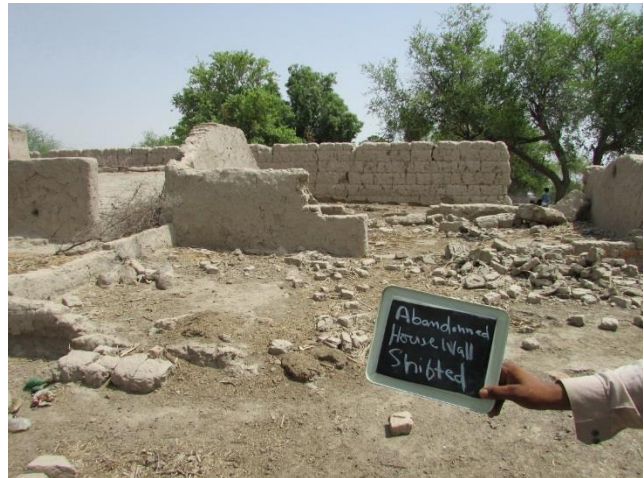
Figure 26: Abandoned House at Spur Extension
