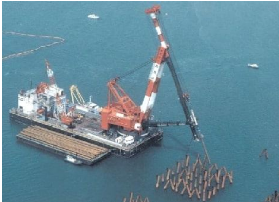
Figure 2.7: Floating Pile Driving Frame through Barge
