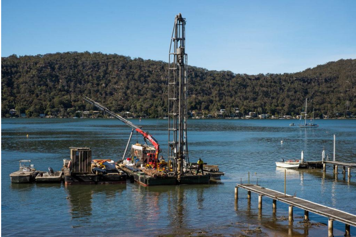
Figure 2.8: Pile Driving Frame for Project Requirements
