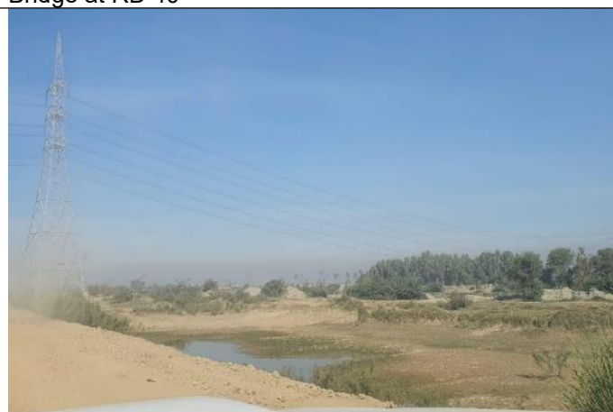
RD 40-50 Rice Canal showing dug-out embankment and utility crossing
