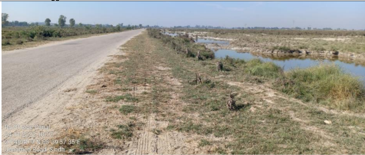
Adjacent access road
