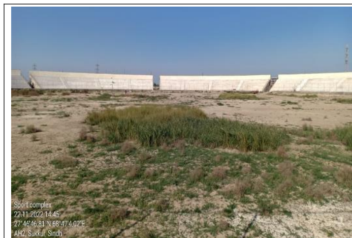
The floor of the stadium to be filled
