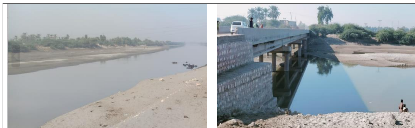
Rice Canal at RD 40 facing left bank / downstream
