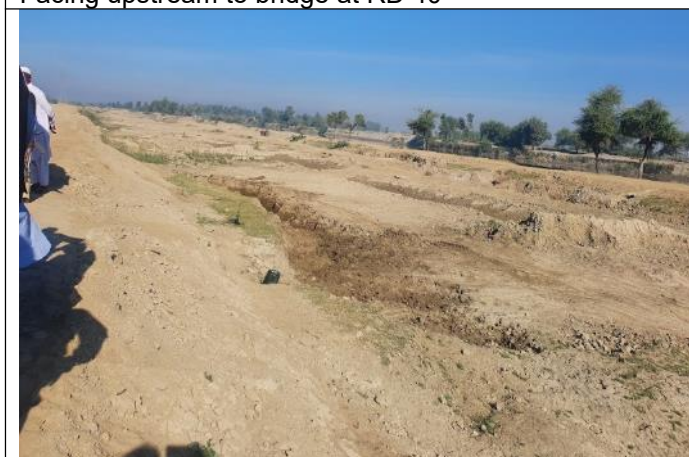
RD 40-50 Rice Canal showing dug-out embankment and utility crossing
