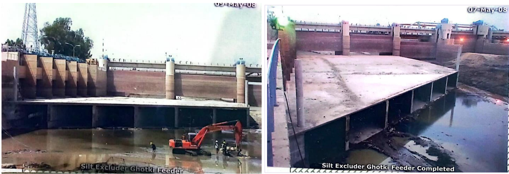
Figure 1.4: General arrangement of the existing silt excluder (photographic views)
