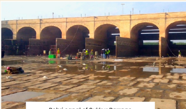
Rohri canal of Sukkur Barrage
