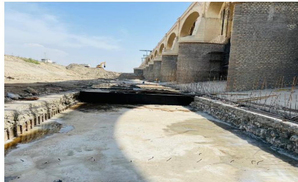
Settled apron at U/S of bays 15 to 17 repaired
