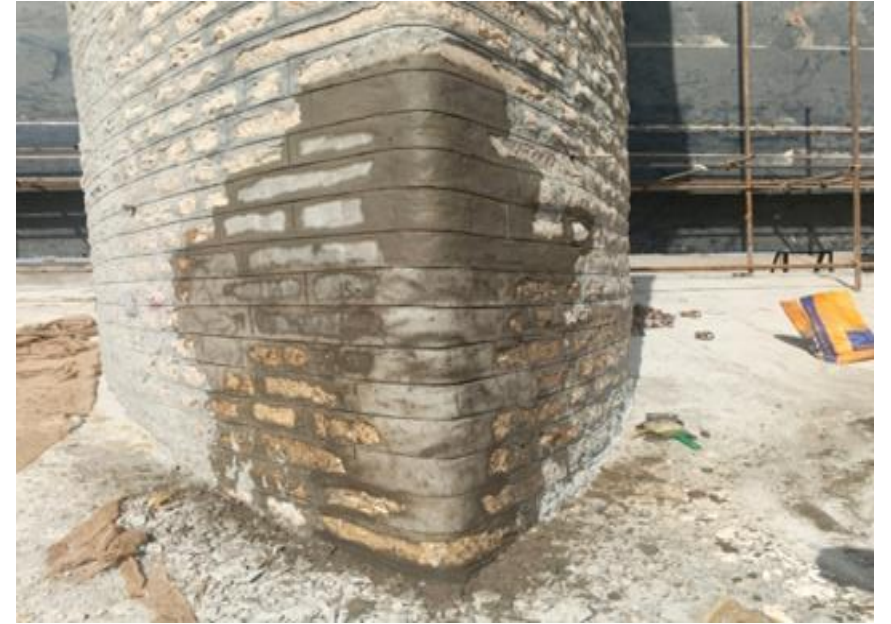
Civil repair for damaged areas
