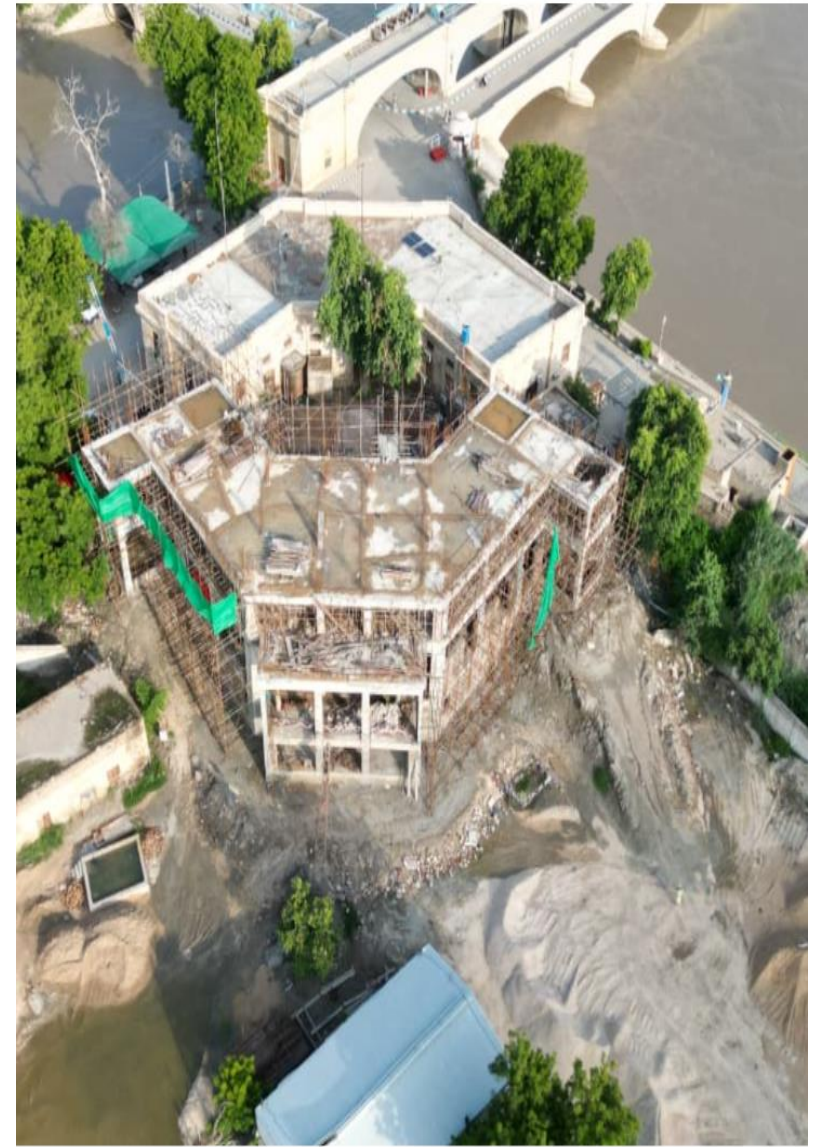
B4 building for Irrigation- finishing works
