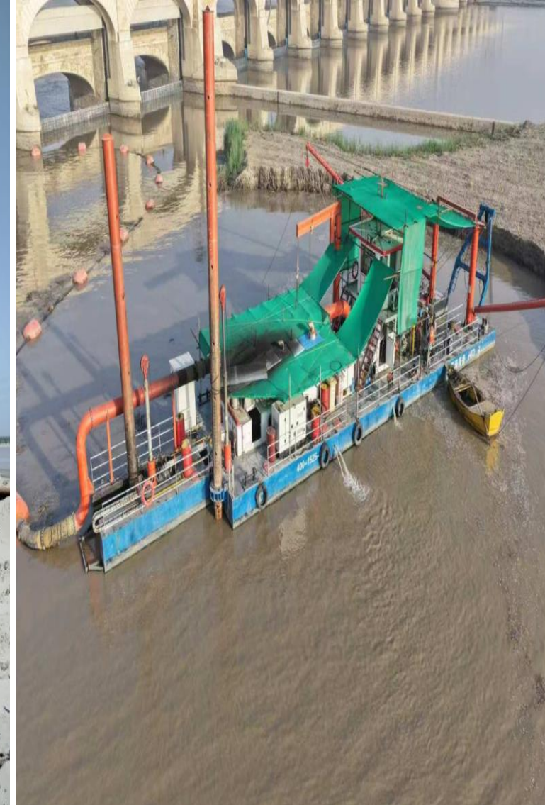
Dredger at Left Pocket
