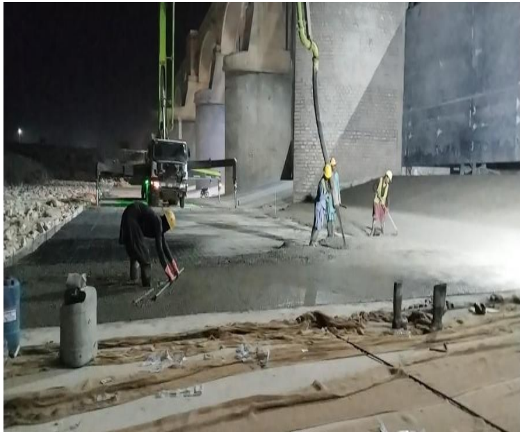
Overlay concreting at apron
