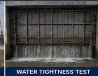
WATER TIGHTNESS TEST
