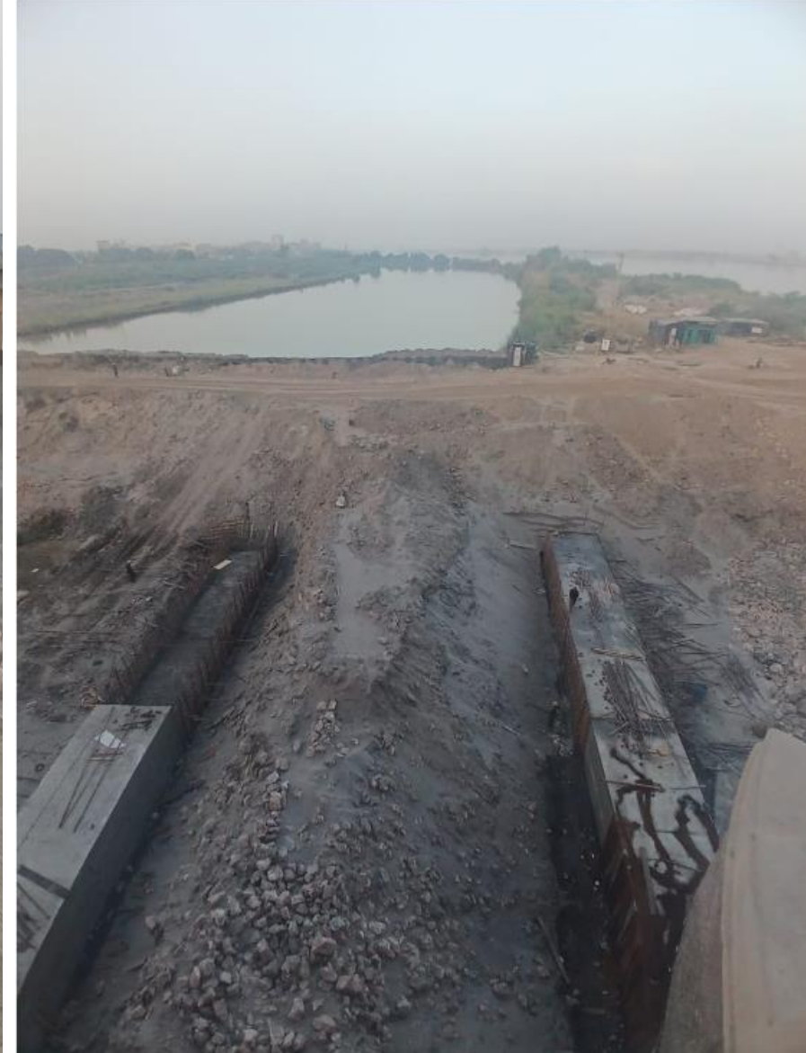
Bay 23 & 24 - Construction of new low height wall
