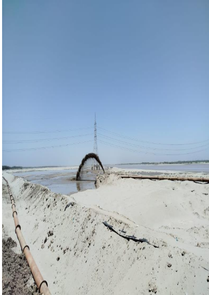
Dredging Pipeline disposal site at
