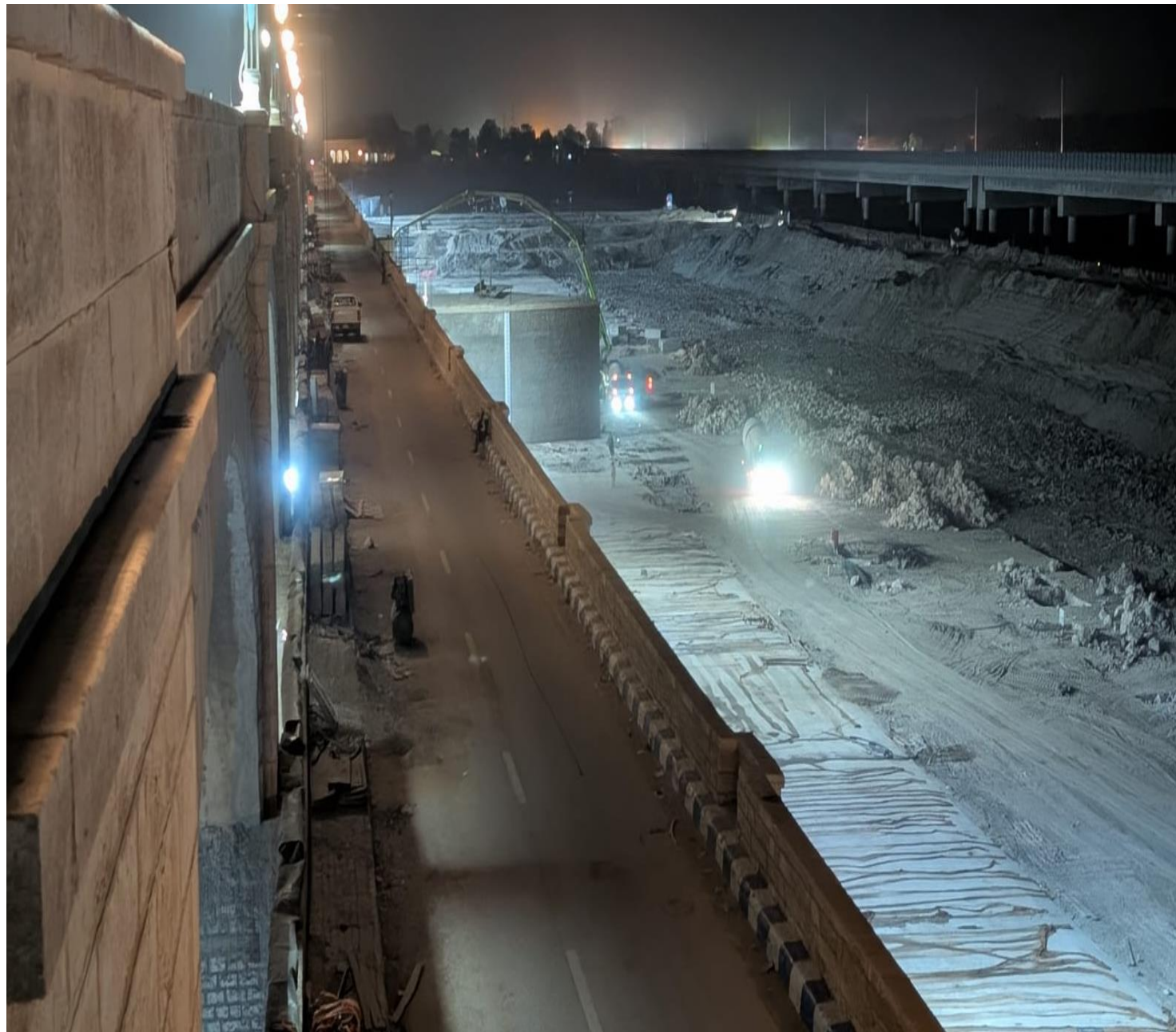
Cofferdam (covering 30 bays D/S side)
