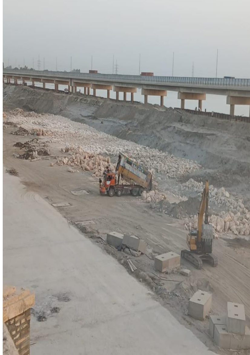
Rip-rap (stone dumping) D/S as per Artelia Model Study
